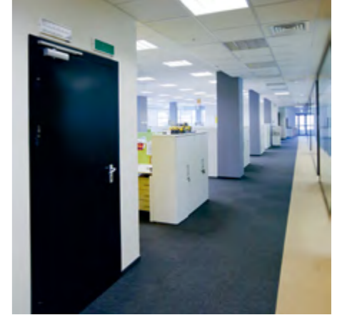
Full metal doors, perimeter door fireproof seal.
