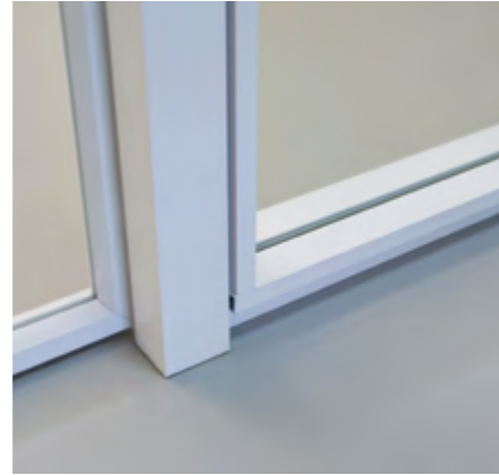
C Junction of a single-glass wall to the floor
