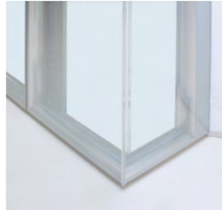
C 90° angle of the solid glass partition
