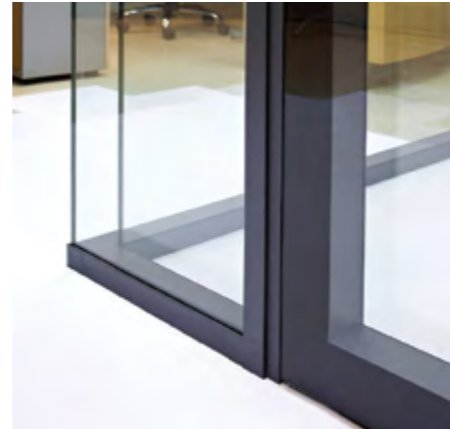
C 90° angle of the solid glass partition
