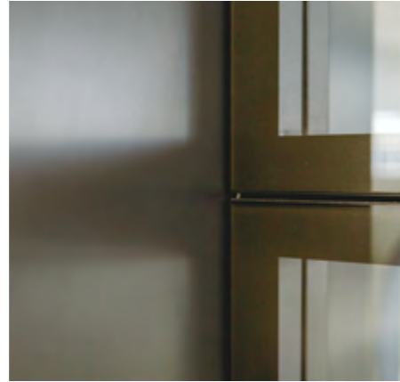
B Junction with a structured double-glass window
